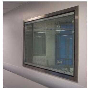
HOLLOW METAL STEEL FIXED WINDOWS
